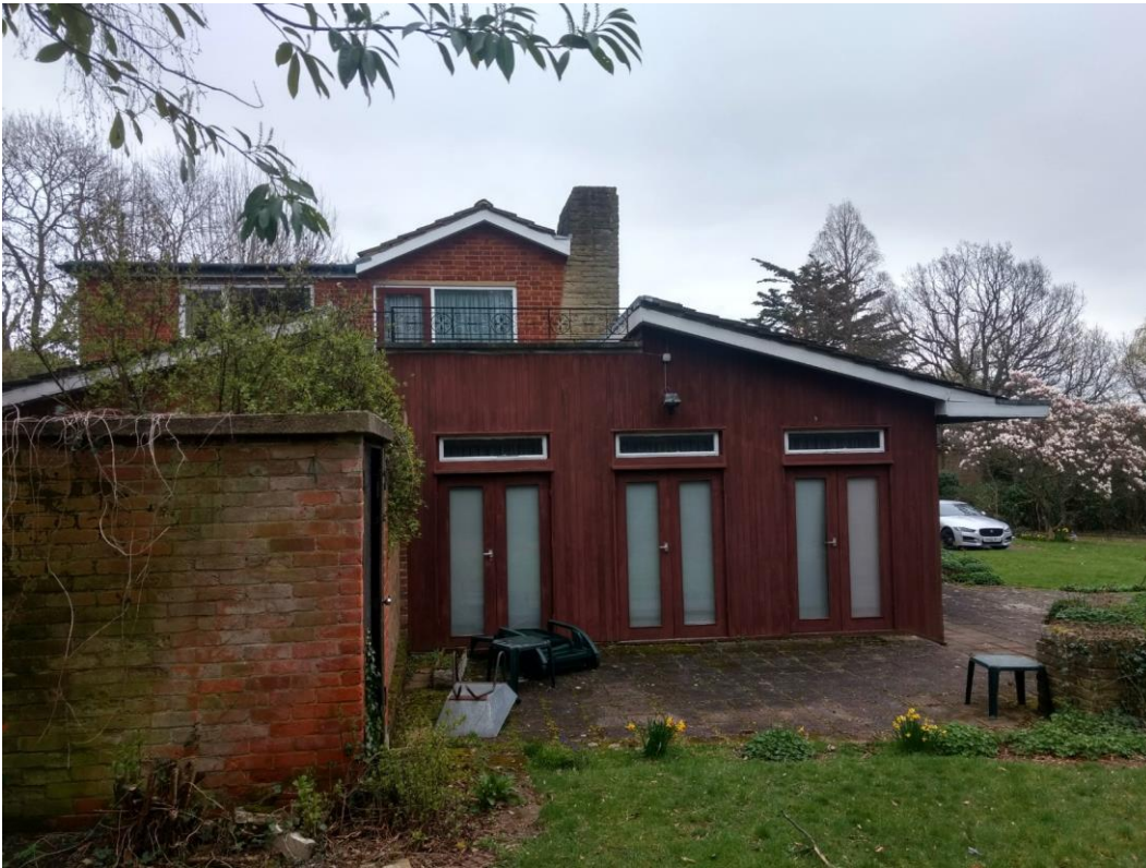
Existing west facing flank wall
