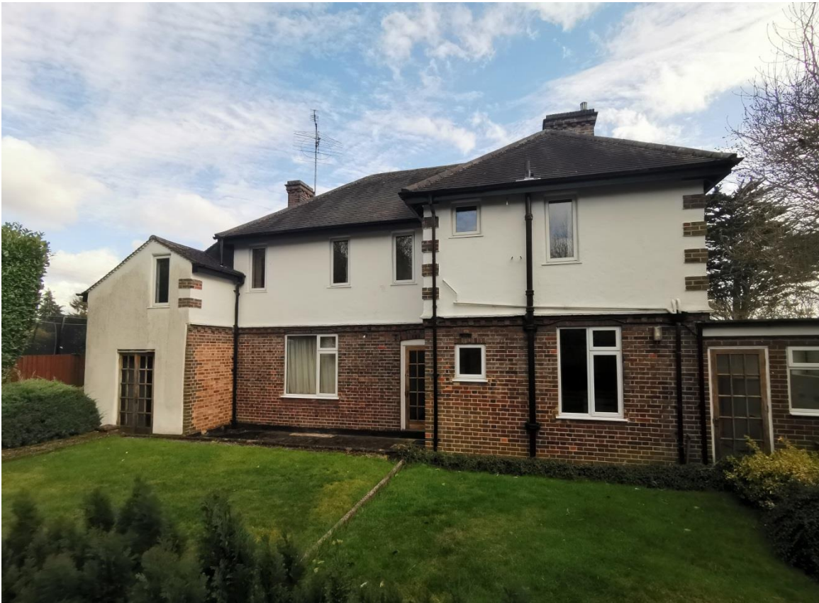
Figure 2 Existing rear elevation
